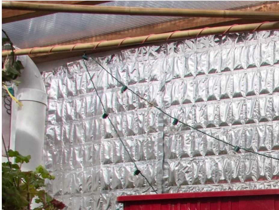
Fig.1 [5] Example of PCM module placement on the interior wall of a solar greenhouse. Reflective packets filled with PCM (paraffin-based mixture) absorb solar heat during the day and reduce heat loss through the wall at night, thereby increasing nighttime air temperature.
